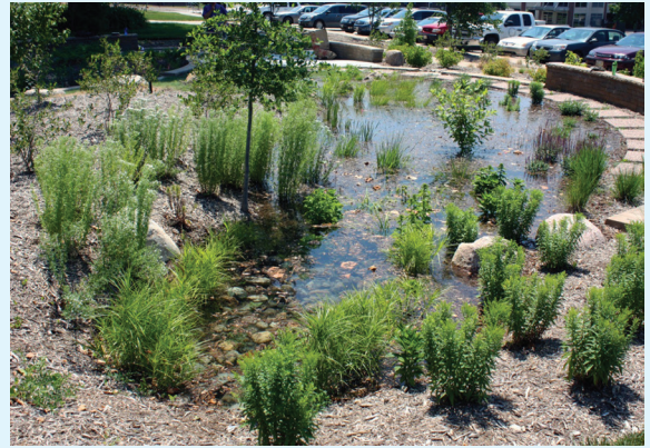
Figure 2. A bioretention garden after a rainstorm. Bioretention gardens capture and filter runoff and let it soak into the soil, usually within 24 to 48 hours.
