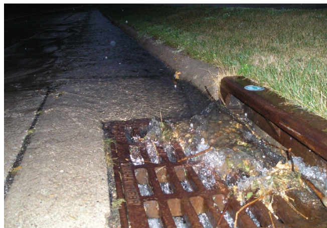
Figure 1. Stormwater runoff flowing into a storm drain. From here it flows directly to a nearby stream, river, or other surface water body.
